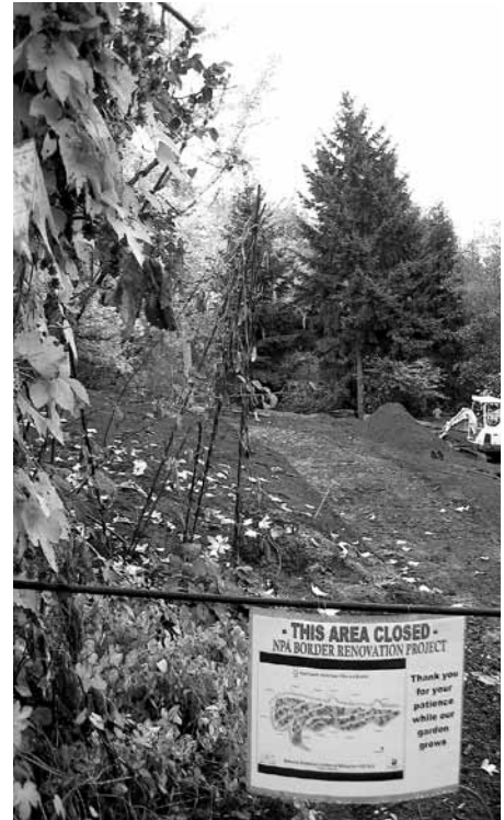
South Border under construction
